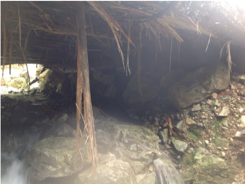
Left Bank Abutment when facing downstream
