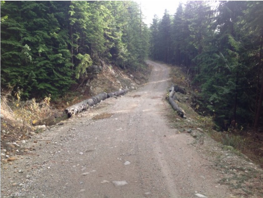
Approach from Right Bank when facing downstream
