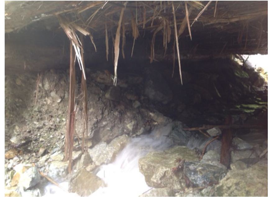
Right Bank Abutment when facing downstream
